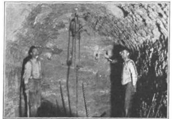
TUNNEL FACE SHOWING USE OF COAL AUGERS
